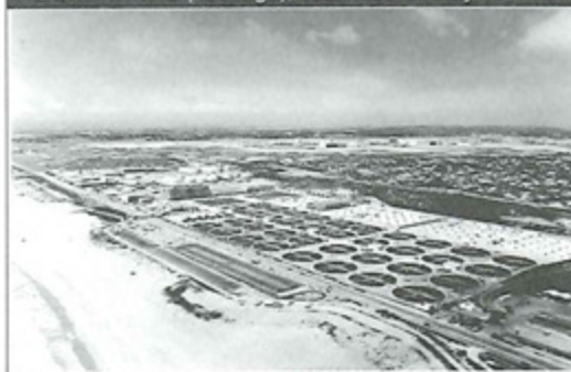
City of Los Angeles Hyperion Wastewater Treatment Plant 1.7 M m^3/d (450 mgd), dedicated on May 15, 1999
